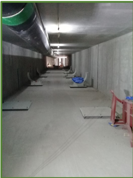
Pipe Supports Installation & Pipe Laying in Tunnel (JODC Project)
