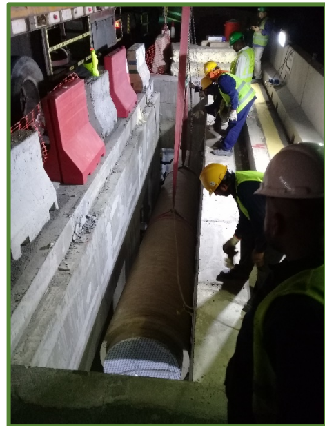
Pipe Supports Installation & Pipe Laying in Tunnel (JODC Project)
