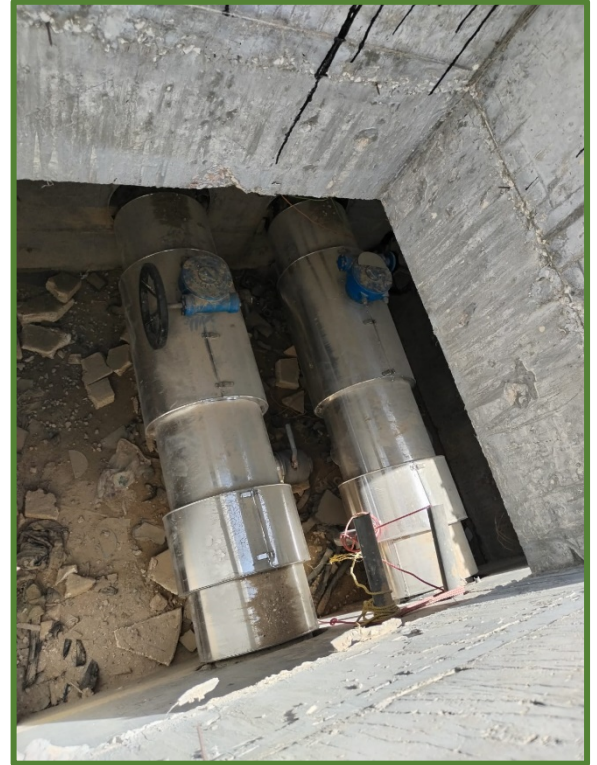
Tie-In with Insulated Pipes
